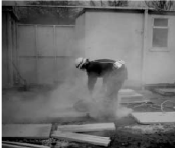
(a) Figure 2 Slab cutting with main supply water system: (a) without control; (b) with control
