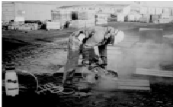
(a) Figure 1 Slab cutting with pressurised portable tank system: (a) without control; (b) with control
