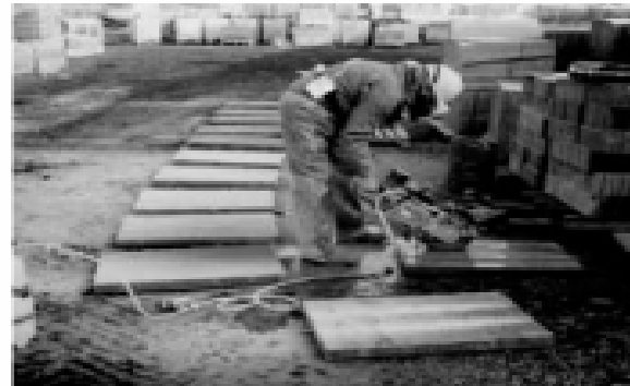
(a) Figure 1 Slab cutting with pressurised portable tank system: (a) without control; (b) with control
